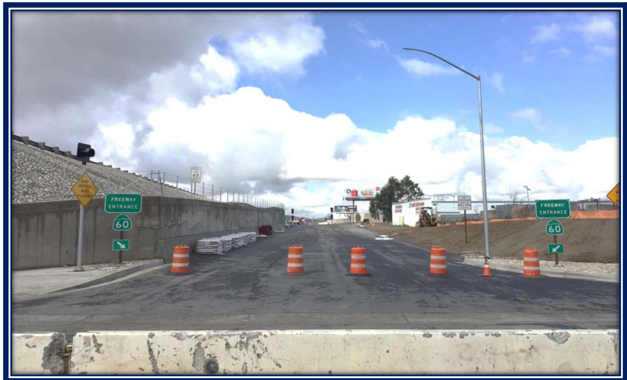
Lemon Avenue – 57/60 Freeway on and off ramps construction
