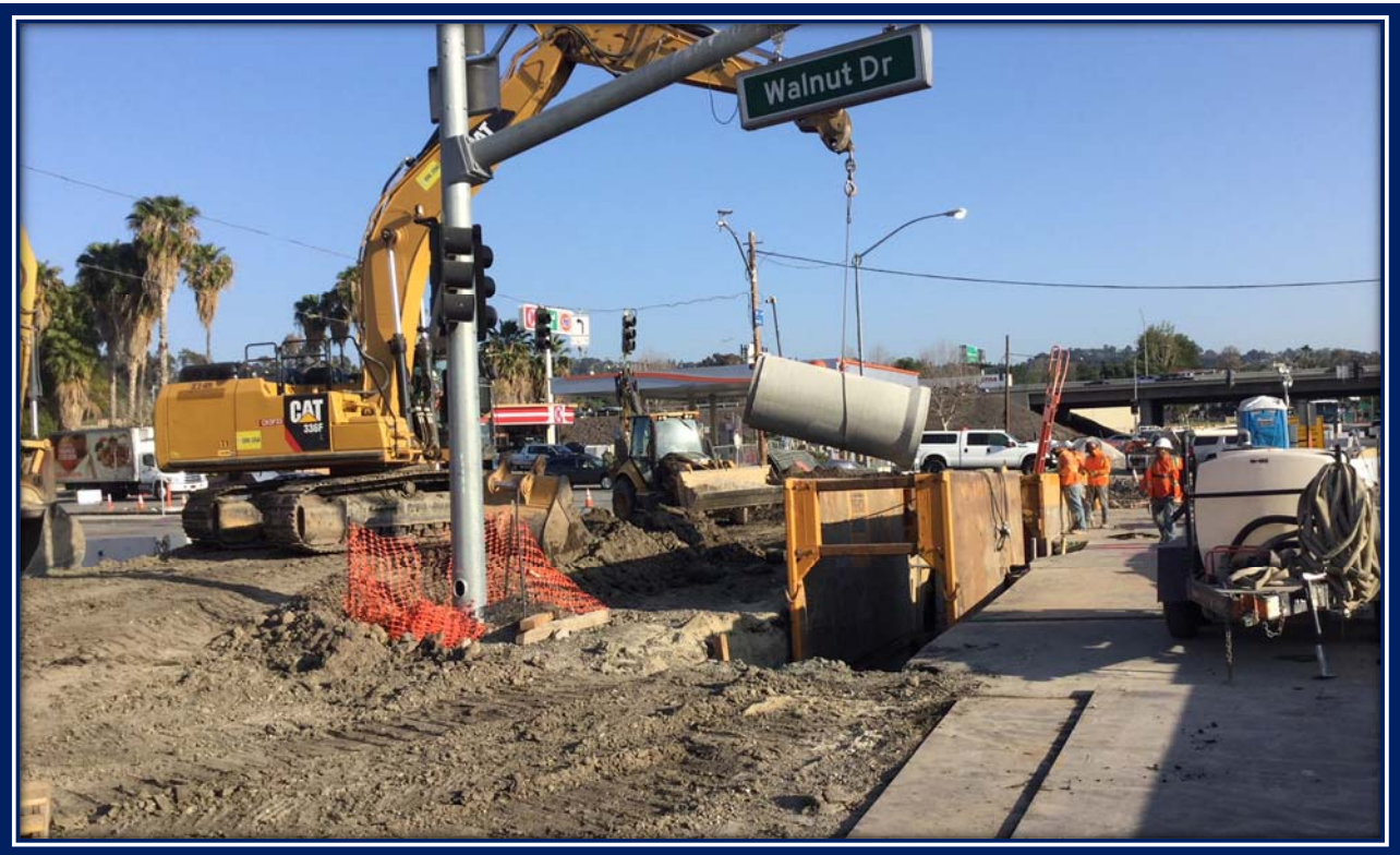
Fairway Drive – Storm Drain construction
