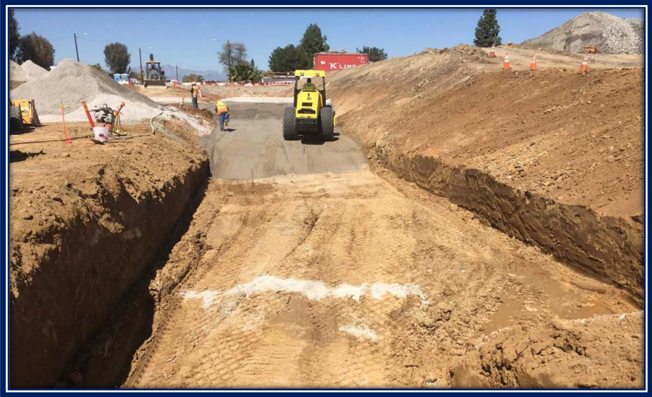
Fullerton Road – Retaining wall excavation
