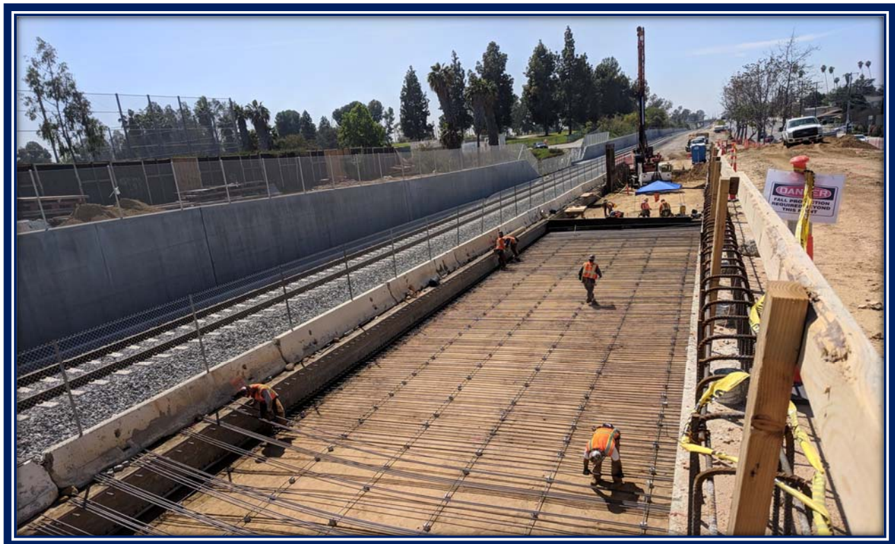
San Gabriel Trench – Bridge deck construction
