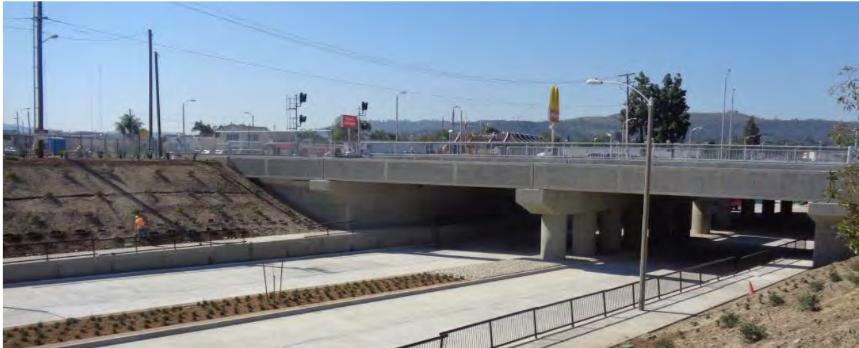
Puente Avenue (Opened to traffic April 2018)
