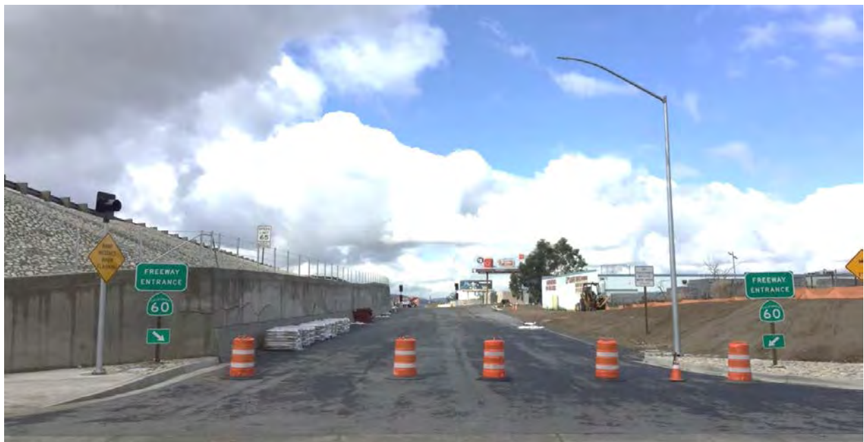
Lemon Avenue (57/60 Freeway On and Off Ramps Construction)
