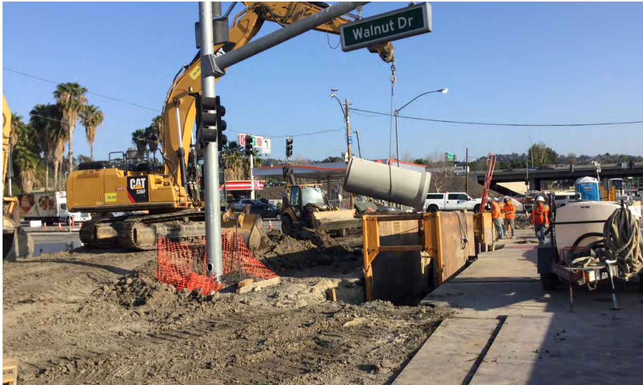
Fairway Drive (Storm Drain Construction)
