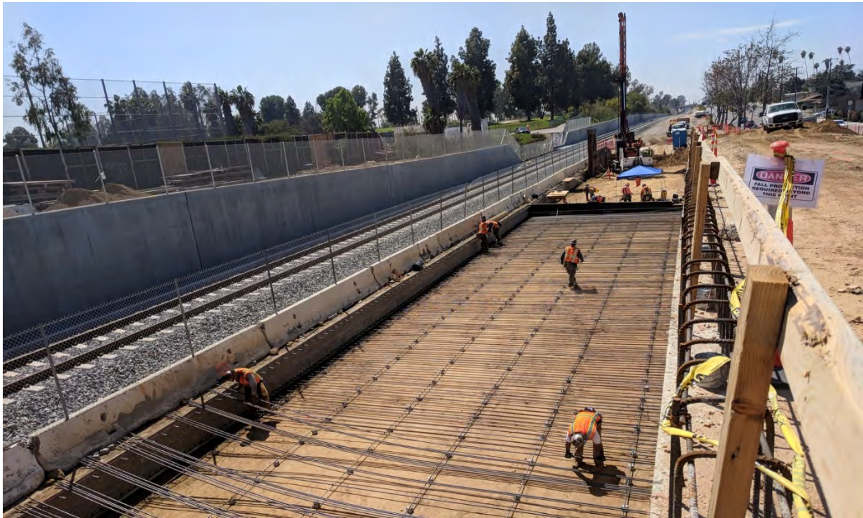
San Gabriel Trench (Bridge Deck Construction)
