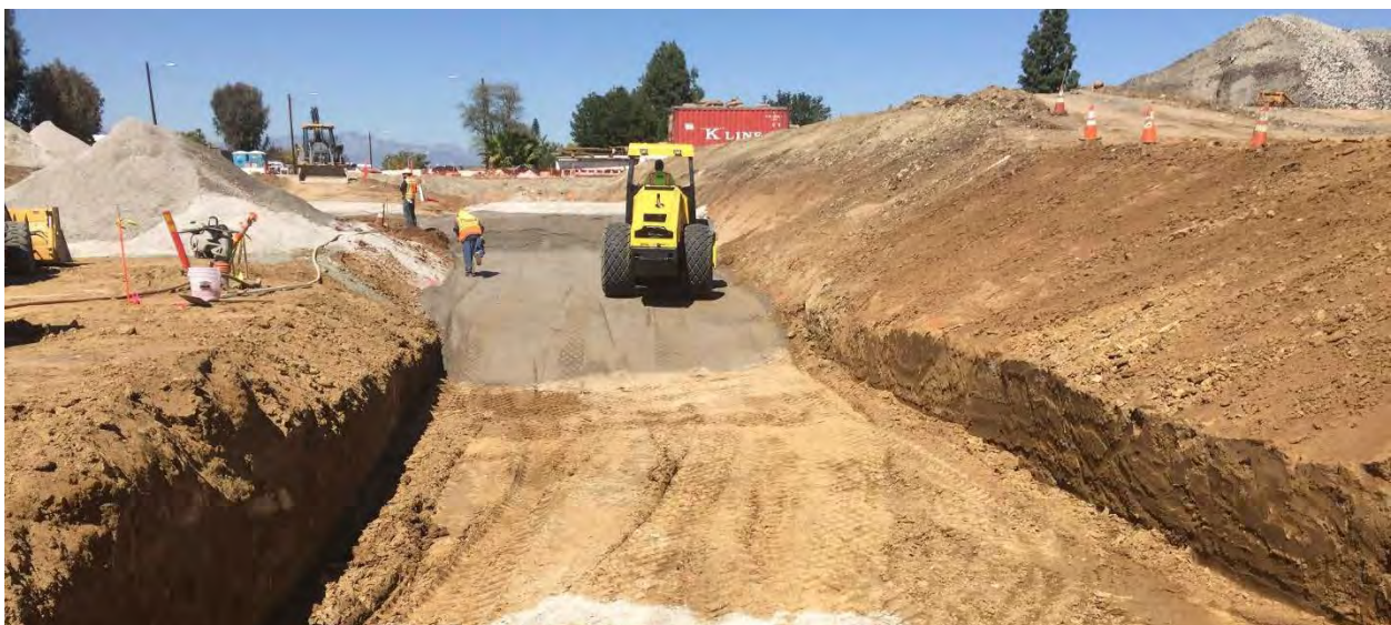
Fullerton Road (Retaining Wall Excavation)
