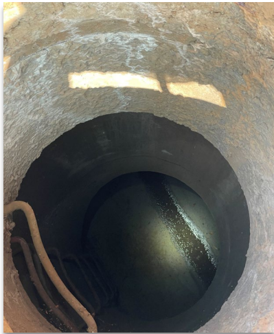
Manhole on Figueroa St. at N. Avenue 53
