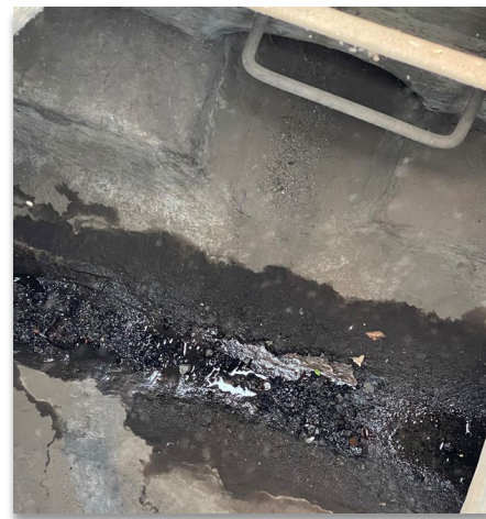
Manhole on N. Avenue 61 at Figueroa St.
