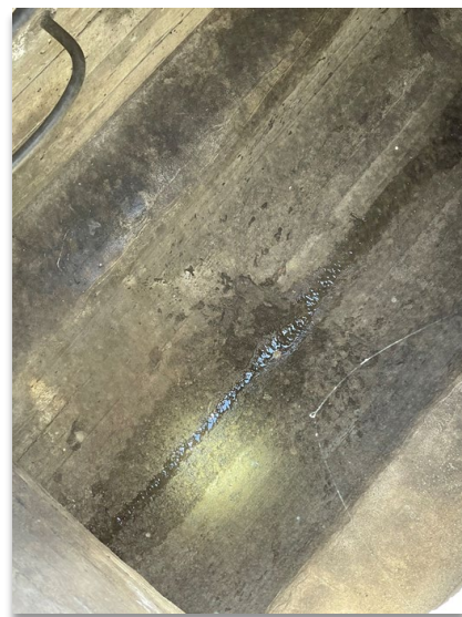
Manhole on N. Avenue 56 at Figueroa St.
