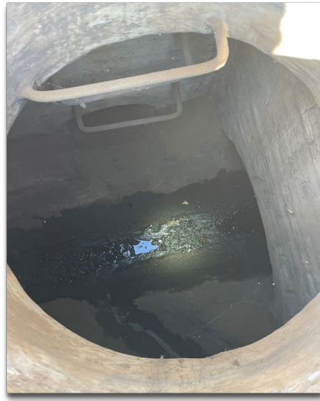
Manhole on N. Avenue 61 at Figueroa St.
