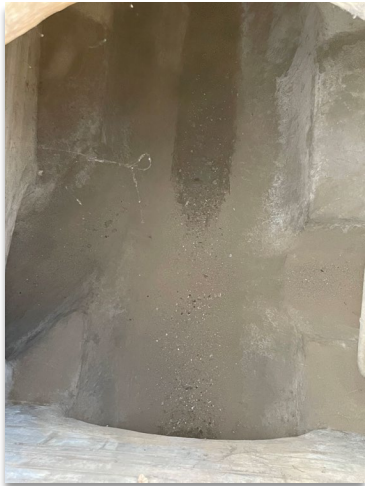
Site #5 (Manhole on N. Avenue 61 at Figueroa St.)
