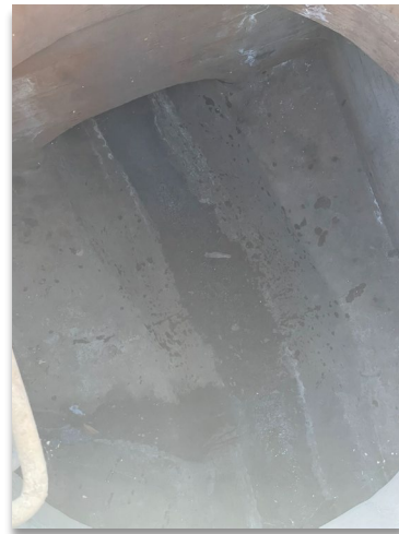
Site #4 (Manhole on Figueroa St. at N. Avenue 61)
