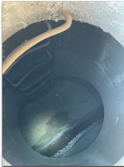
Manhole on Figueroa St. at N. Avenue 53
