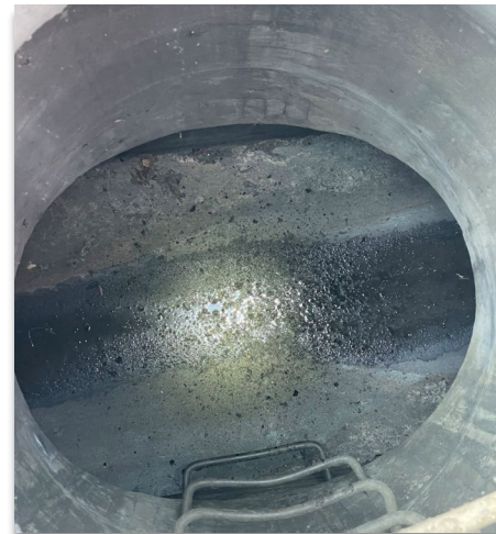
Manhole on Figueroa St. at N. Avenue 57
