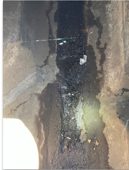
Manhole on N. Avenue 61 at Figueroa St.
