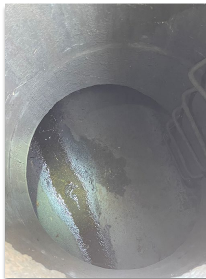
Manhole on Figueroa St. at N. Avenue 53
