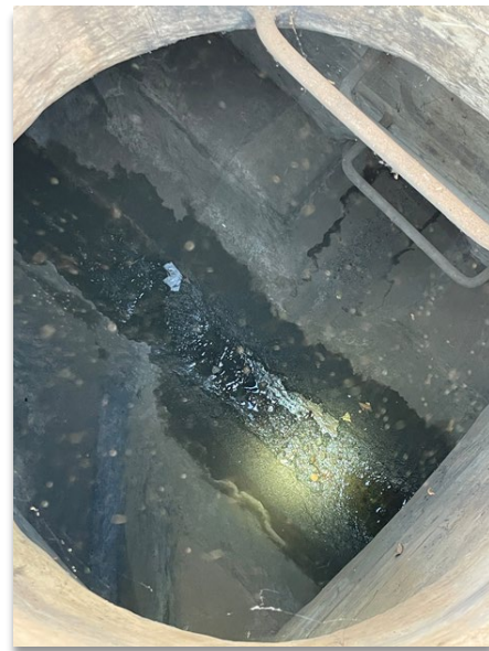
Manhole on N. Avenue 61 at Figueroa St.
