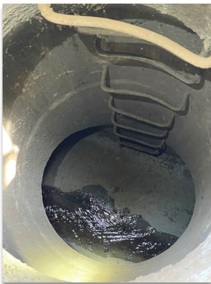
Manhole on Figueroa St. at N. Avenue 53
