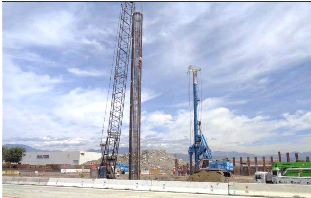
CAST IN DRILL HOLE PILE DRIVING – PUENTE AVENUE GRADE SEPARATION PROJECT – CITY OF INDUSTRY
