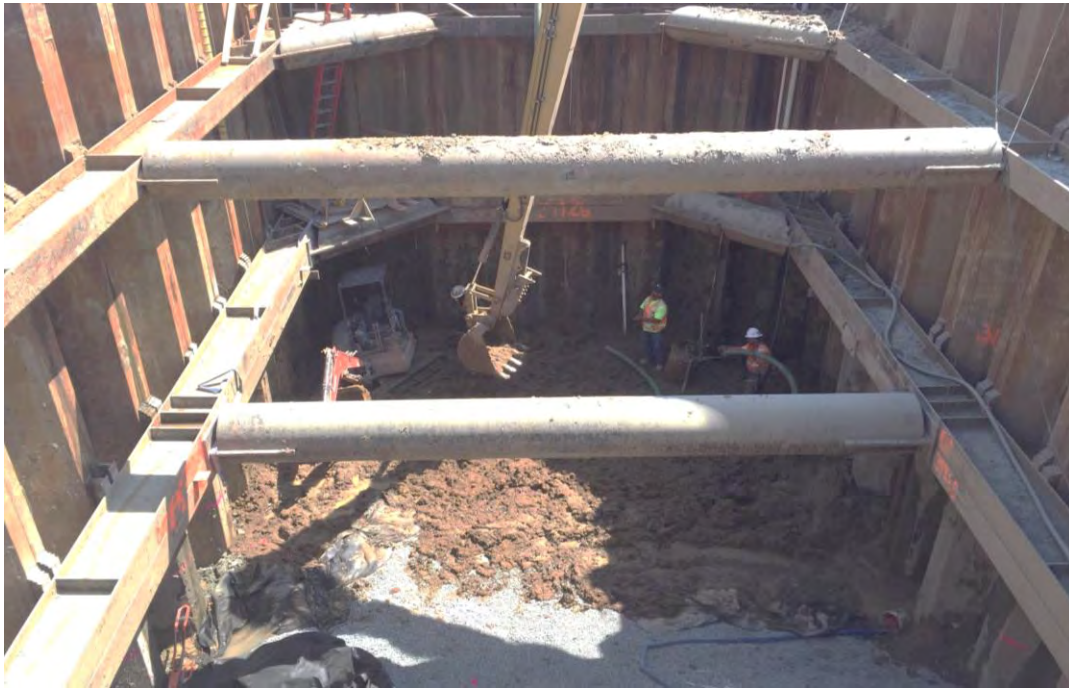
PUMP STATION EXCAVATION – FULLERTON ROAD GRADE SEPARATION PROJECT – CITY OF INDUSTRY
