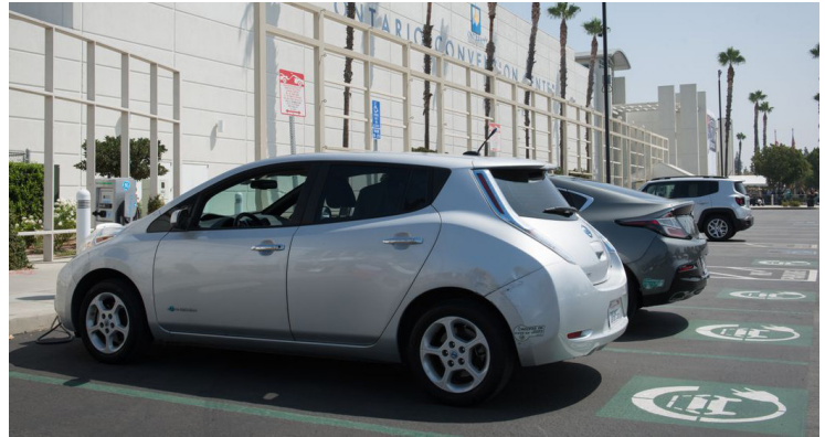
Through the Charge Ready program, the city of Ontario installed more than 45 EV chargers throughout the city, including at the Ontario Convention Center (pictured). Photo: Paul Griffo
