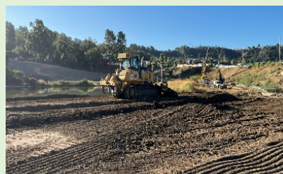
Grading new fairways, bunkers, and greens
