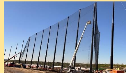
Netting strung on boundary poles
