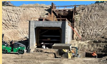
Cart tunnel under construction
