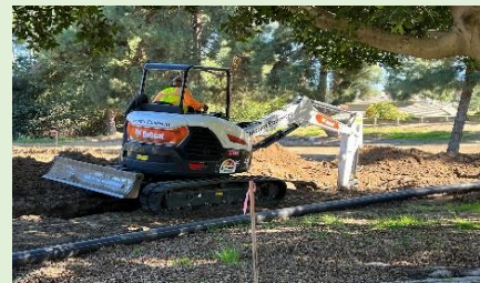
New irrigation pipe installed
