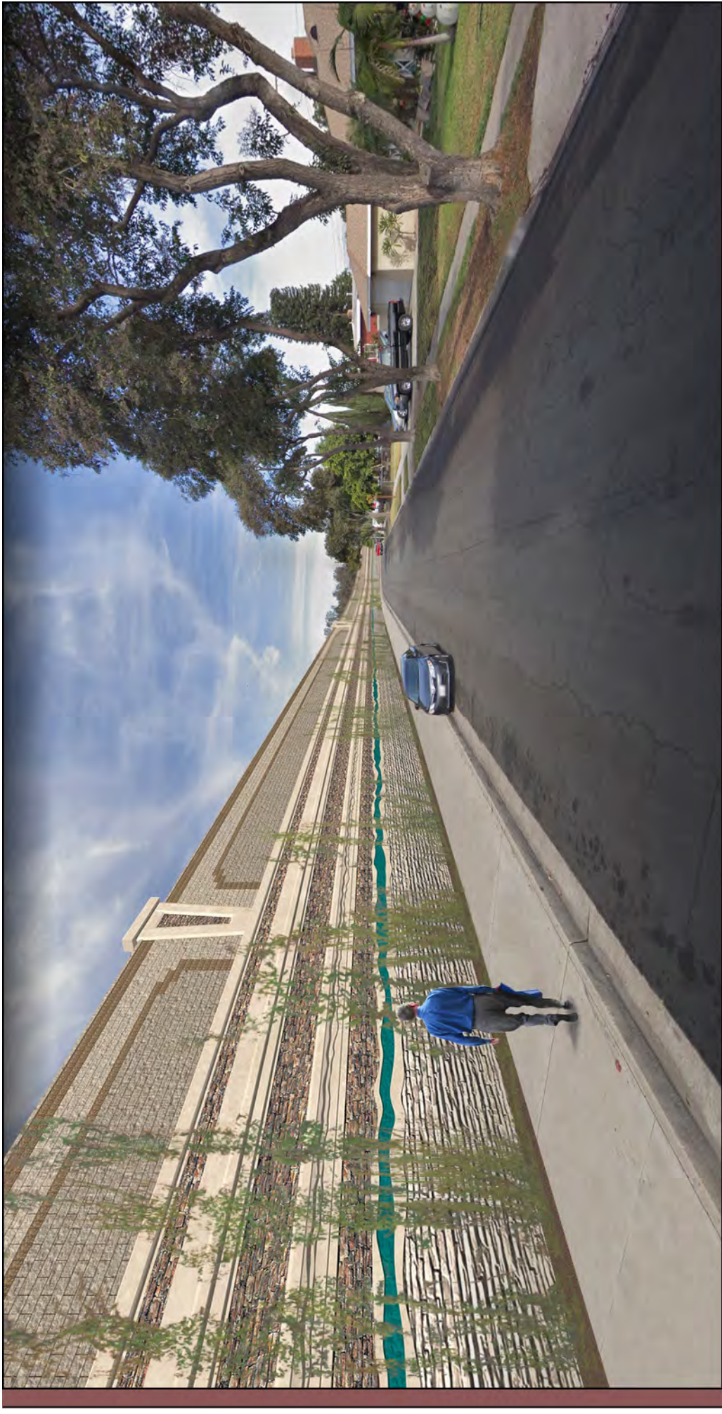
DRystack TEXTURE TO MATCH FITZGERALD PATTERN #17911 - 1 1/2" RELIEF SAN DIEGO DRystack TEXTURE PAINT COLORS TO MATCH #'S 30117, 30215, 36251, AND 37722 OF FED-STD-595
