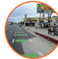
COLOR PAVEMENT TREATMENT Green Conflict Striping
