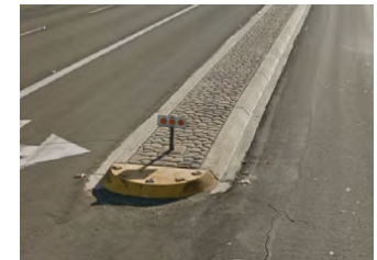
Concrete separator for access management (2')
