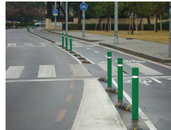
Heavy bollards for car/bike separator, separated bike lane
